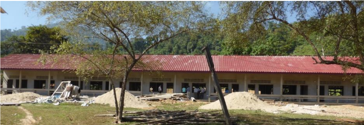
Photo 3: School in construction in Phadai Village, Bolikhan District, Bolikhamxay Province
